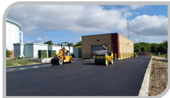
SAWS Maltsberger Pump Station Improvements – existing 5 million gallon ground storage tank rehabilitated and new electrical building completed to improve system reliability.
