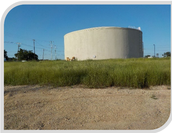
Intermediate Pump Station 1 – 4 Million Gallon ground storage tank.
