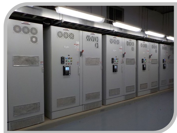
Motor Control Center for the four large pumps at the High Service Pump Station that move water to San Antonio.
