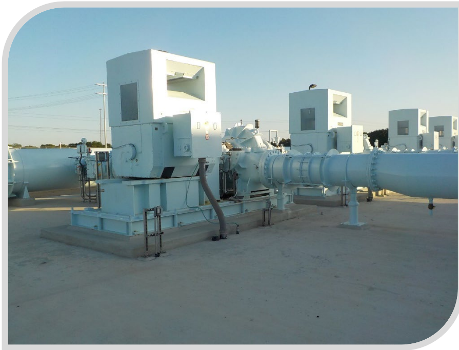
Intermediate Pump Station 1 near Elgin. One of two booster pump stations that keep water moving to San Antonio. Houses a four million gallon tank and four large pumps. Each pump is capable of delivering 17 million gallons per day.
