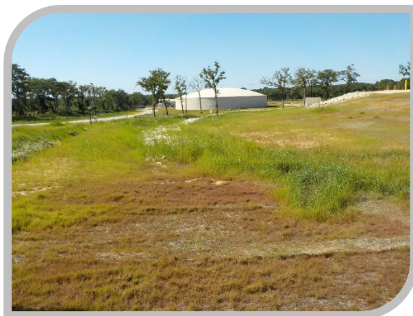
The High Service Pump Station in Bureson County located next to the well field. Houses a four million gallon tank, cooling tower, disinfection equipment, and four large pumps that send treated water to San Antonio.
