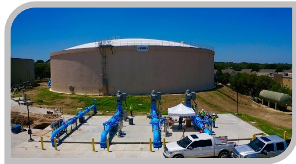
SAWS Bitters Pump Station Improvements – new 5 million gallon ground storage tank and 30 million gallons per day pump station put in service in April 2020.
