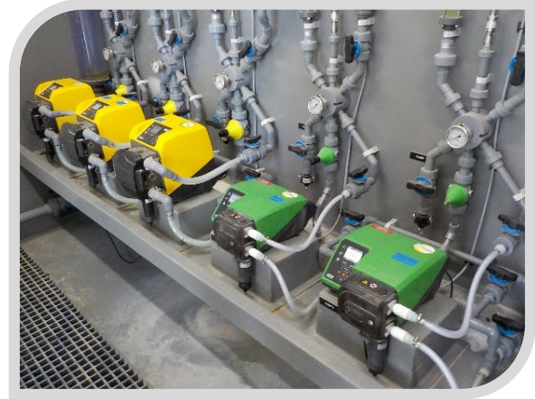
High service pump station chemical disinfection feed pumps.
