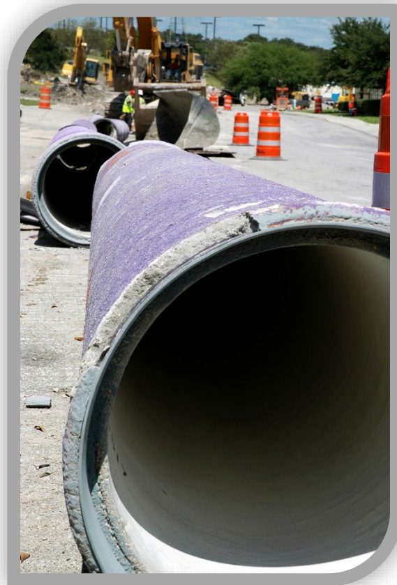
Recycled water pipes at a construction site.
