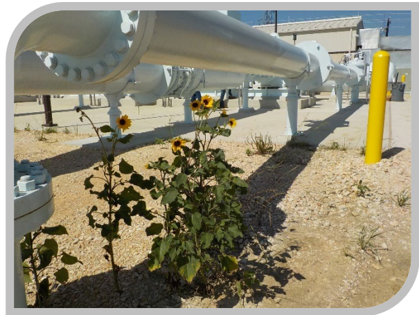
Intermediate Pump Station 2 near Seguin. One of two booster pump stations that keep water moving to San Antonio. Houses a four million gallon tank and four large pumps.
