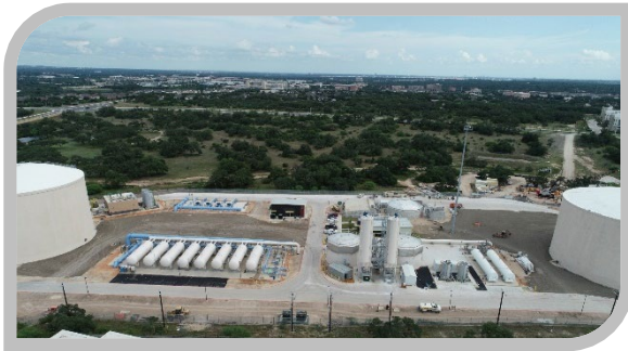
SAWS Agua Vista Station – water conditioning facility at point of delivery; Phase 1 completed on January 16, 2020 and Phase 2 completed on April 15, 2020.
