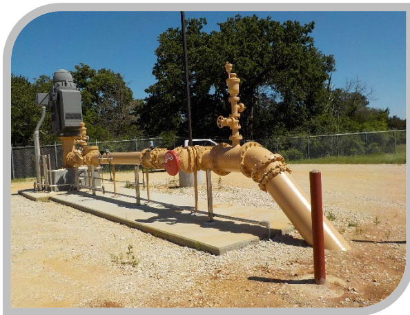
VR Simsboro Well Pump, one of nine – yields approximately 3,000 gallons per minute.
