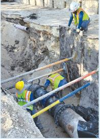
water leak detection and repairs, to reduce water loss within the SAWS distribution system.
