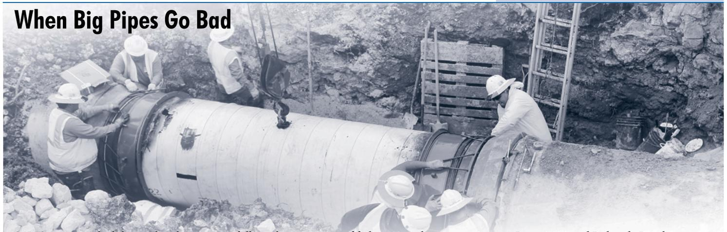
SAWS crews worked day and night to successfully replace a section of failing 48-inch water main near Loop 1604 and Bulverde Road on the city's Northeast Side, Jan. 9-10, 2016. Thanks to careful planning, only about 650 homes were without water service during the repair. The operation was also carried out over the weekend to minimize the outage's impact to residents' work and school schedules.
