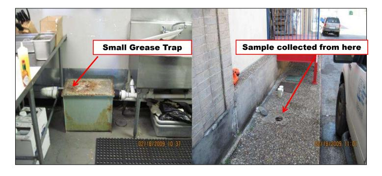
Small grease traps are required to maintain cleaning logs or manifests
