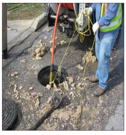
Without pretreatment, FOG accumulates in the sewer main and causes SSOs
