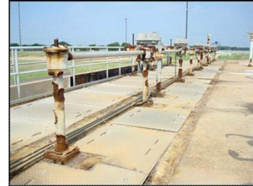
Photo 6 – Pre-aeration Tank Slide Gates
