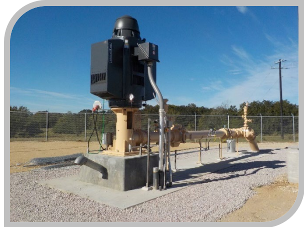
Tunnel shaft piping for crossing the San Marcos River. Completed Simsboro Aquifer 900 hp production well.
