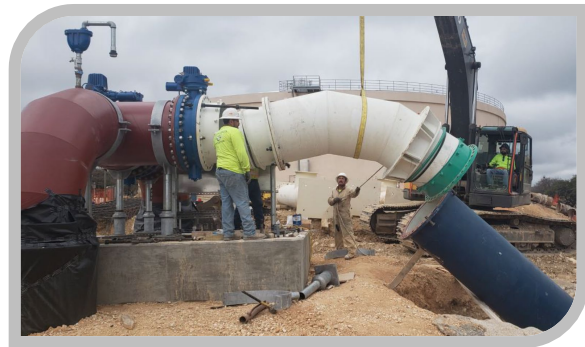
SAWS Bitters Pump Station Improvements – control valve piping installation to facilitate integration of Vista Ridge water.
