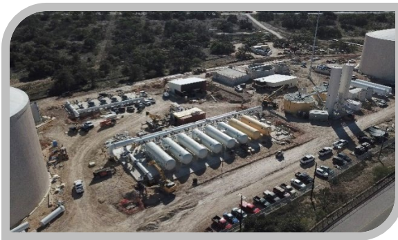
SAWS Agua Vista Station – water conditioning facility at point of delivery; Phase 1 nearing completion to accept Vista Ridge water during performance testing.
