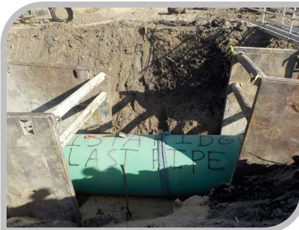
The final segment of 60-inch steel pipe was installed September 25 th in Guadalupe County between New Braunfels and Seguin.
