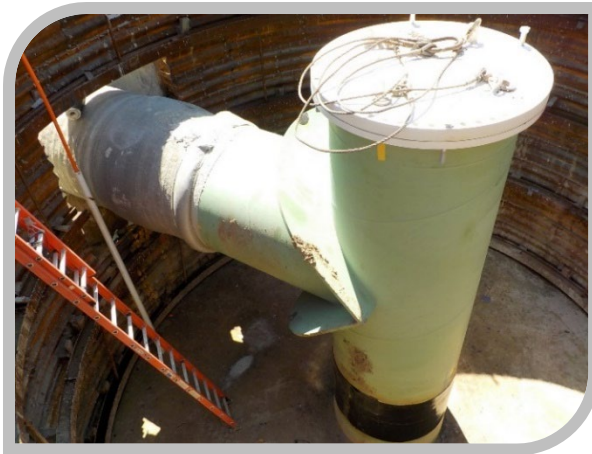
Tunnel shaft piping for crossing the San Marcos River. Completed Simsboro Aquifer 900 hp production well.
