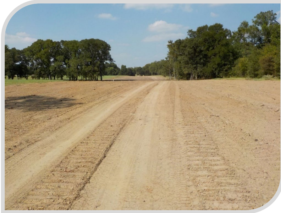
Site restoration work in Bureson County which includes placing of top soil and reseeding. The site is reseeded with a blend of native herbaceous seed mixture for surface restoration of native pastures areas which includes: Little Bluestem, Big Bluestem, Switchgrass, Sideoats Grama and Buffalograss among others.
