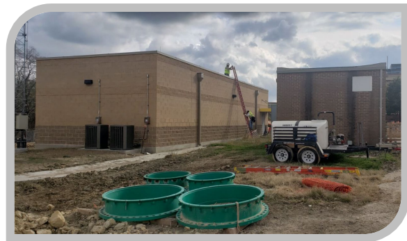
SAWS Maltsberger Pump Station Improvements – new electrical building nearing completion that will improve system reliability.
