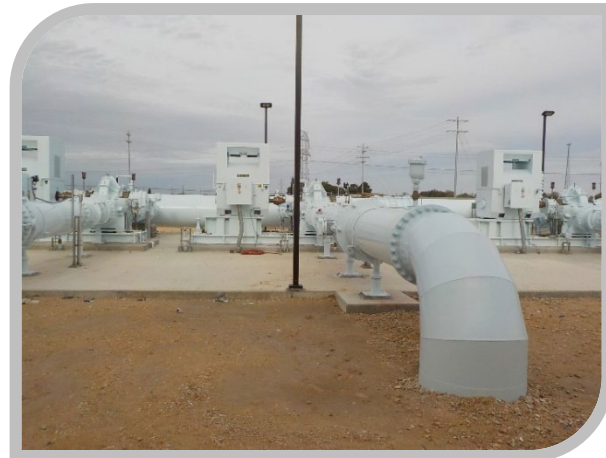
Intermediate Pump Station 1 near Elgin, Texas to maintain flow to Agua Vista Station in San Antonio.
