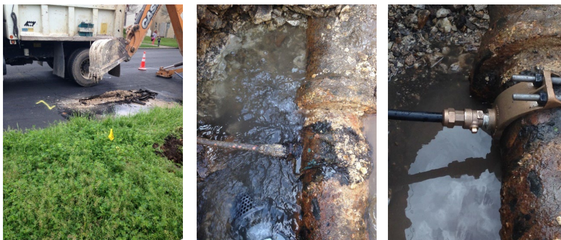
Above: Excavating a hidden leak revealed through proactive planned leak detection
